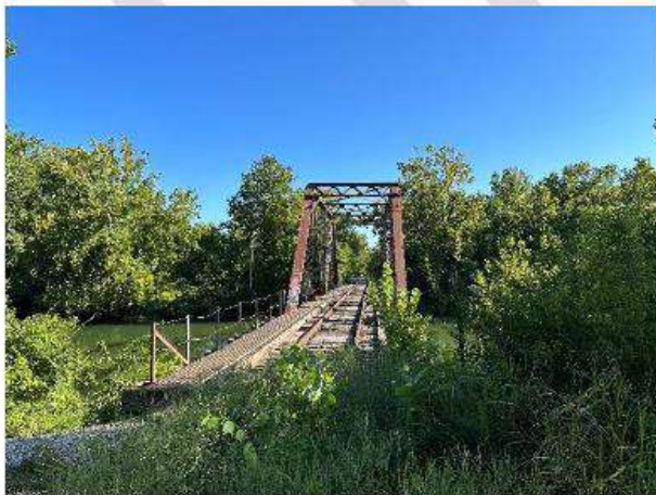
Figure 2: Springfield Lake Bridge
